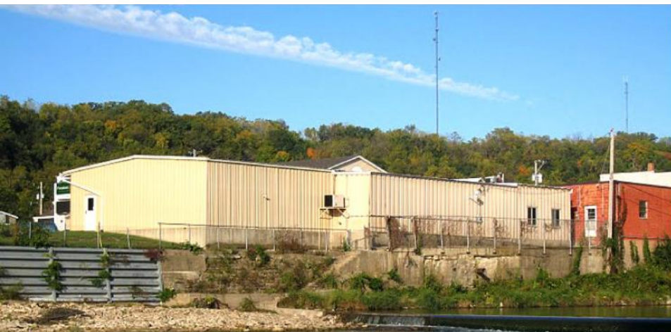
Collapsing river access steps and high floodwalls will be modified in the Spring of 2014 to better connect the community to the new river enhancements.
