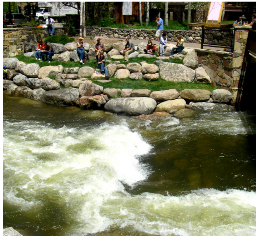
Boulder terracing give spectators a comfortable view and withstood 100 year flooding without damage
