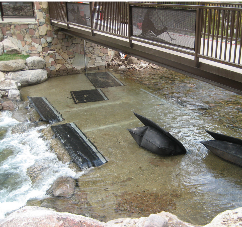
Low flows show inflatable bladders and give access to varied forms of recreation
