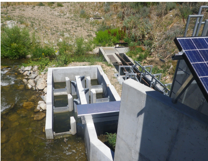
Vertical Slot Fishway from top of structure
