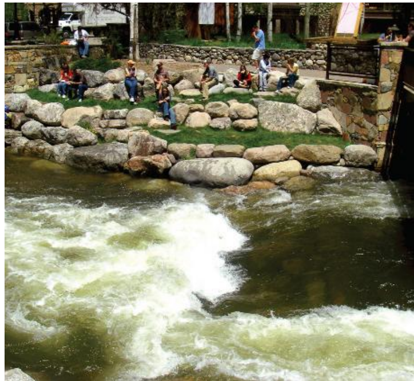
Boulder terracing give spectators a comfortable view and withstood 100 year flooding without damage
