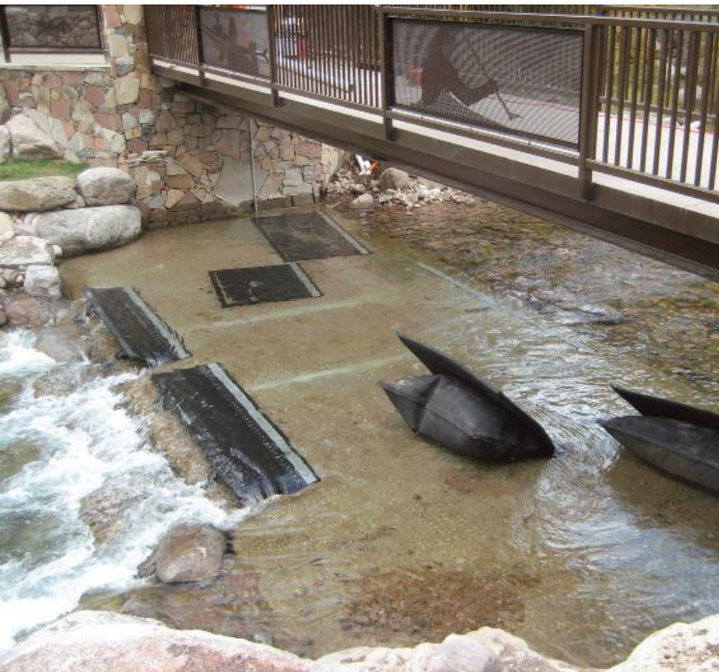
Low flows show inflatable bladders and give access to varied forms of recreation
